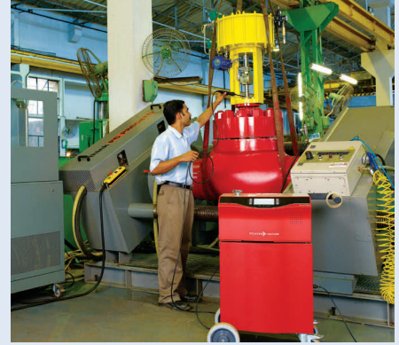
Gland leak measurement for Fugitive Emission testing
