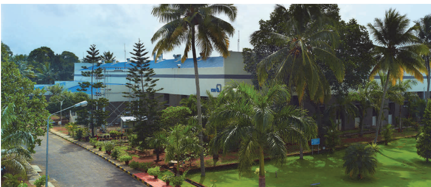
Exterior view of the standard valve manufacturing plant
